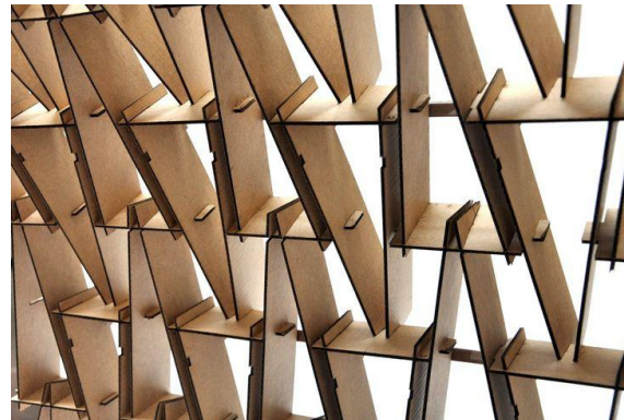
Inter-Lattice Diagrid System
