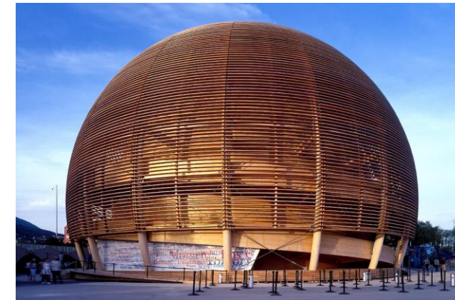
The Globe at CERN, a relocatable exhibition pavilion made entirely of wood.
